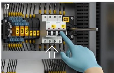
Fig. 13: Check that the magnetothermic switches for disconnection of the fan power supply (Q1) and for disconnection of the auxiliary power supply (Q2) are in the ON position.
