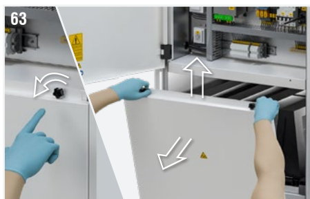
Fig. 63: Unscrew the 2 knobs which keep the rear bottom panel for maintenance access. Lift and then pull you towards to remove the panel.
