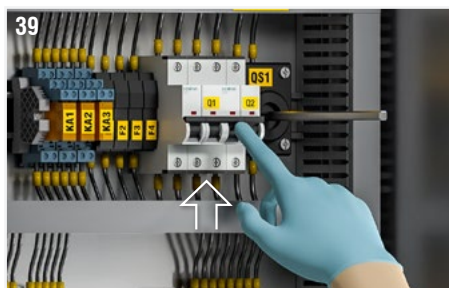
Fig. 39: Check that the magnetothermic switches for disconnection of the fan power supply (Q1) and for disconnection of the auxiliary power supply (Q2) are in the ON position.
