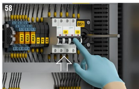
Fig. 58: Check that the magnetothermic switches for disconnection of the fan power supply (Q1) and for disconnection of the auxiliary power supply (Q2) are in the ON position.
