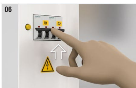
Fig. 6: Check that the magnetothermic switches for disconnection of the fan power supply (Q1) and for disconnection of the auxiliary power supply (Q2) are in the ON position.
