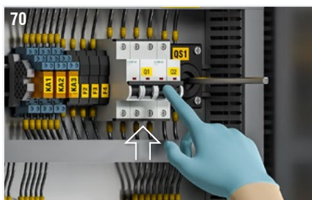
Fig. 70: Check that the magnetothermic switches for disconnection of the fan power supply (Q1) and for disconnection of the auxiliary power supply (Q2) are in the ON position.
