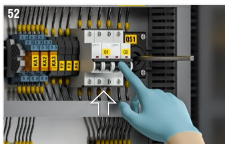
Fig. 52: Check that the magnetothermic switches for disconnection of the fan power supply (Q1) and for disconnection of the auxiliary power supply (Q2) are in the ON position.
