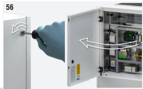
Fig. 56: Use a screwdriver to open the top rear panel.
